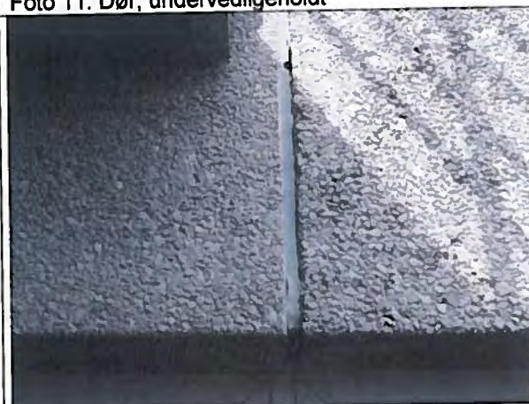
Foto 12: Defekte facadefuger.
