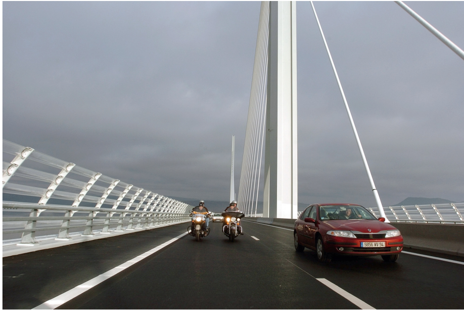
Figure 17. Wind screens on the Millau Bridge in Southern France. The bridge opened December 2004 and is the tallest bridge in the world.
